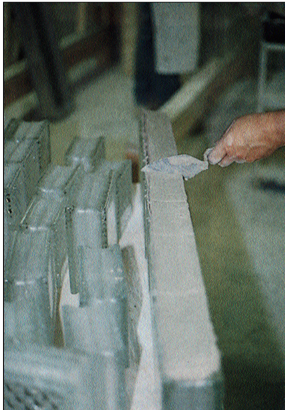
After buttering a row of glass blocks with mortar, the mason slices the mortar at the block edges. A wooden mortar gauge is placed over the dry row of blocks before buttering to ensure a consistent ¼-inch-thick bed of mortar.
