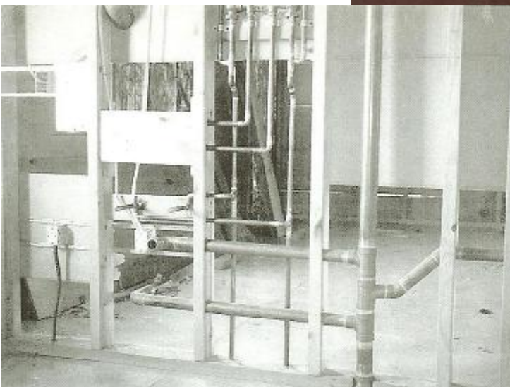
Left: Rough plumbing at Doctor Shultz's house in Chesaning, Michigan. installed by Al Bishop.
